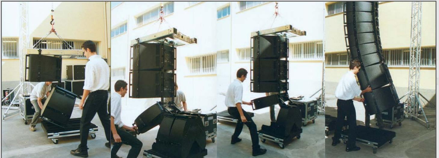
Some stages of the assembly of a Butterfly system made up of eight Hi-Packs and four Low-Packs. This procedure takes just 10 minutes.
